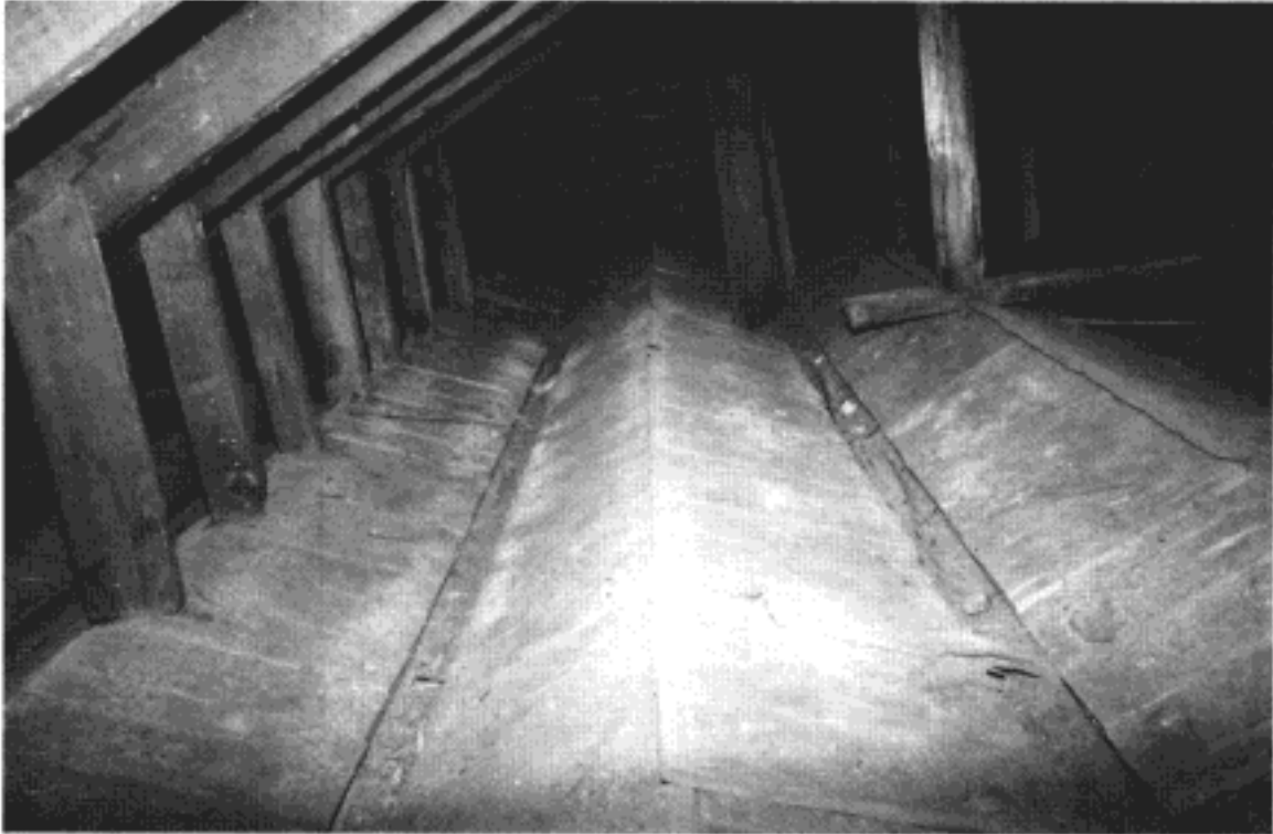
Ridge-and-furrow roof clad with wood boards and tinplate valleys
