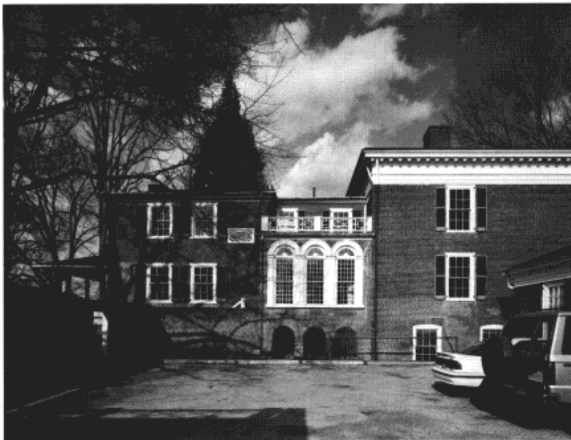
South facade of Pavilion V
