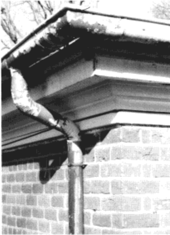
Entablature at southeast corner of rear addition
