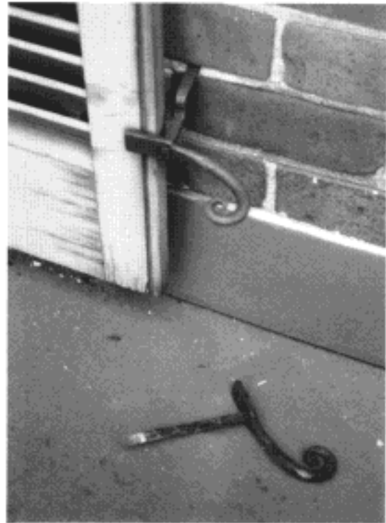
Original wrought-iron holdback for blind
