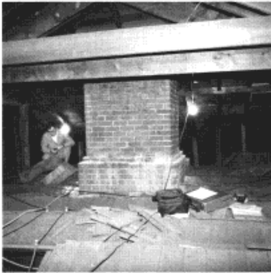
Original chimney stack extended through 1837 hipped roof
