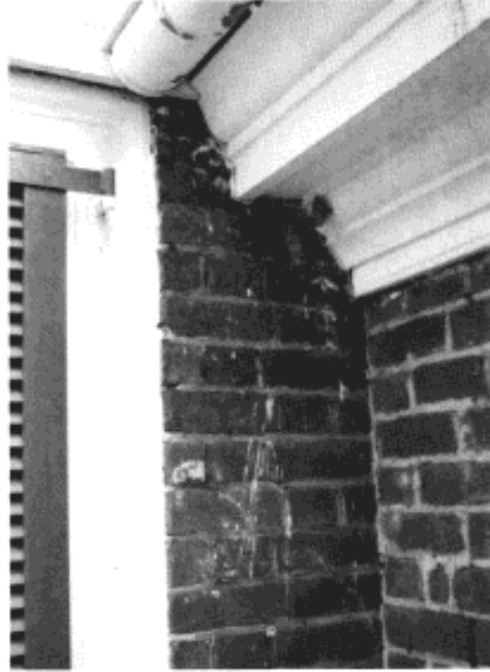
Ghost of original hyphen entablature appears on south face of pavilion
