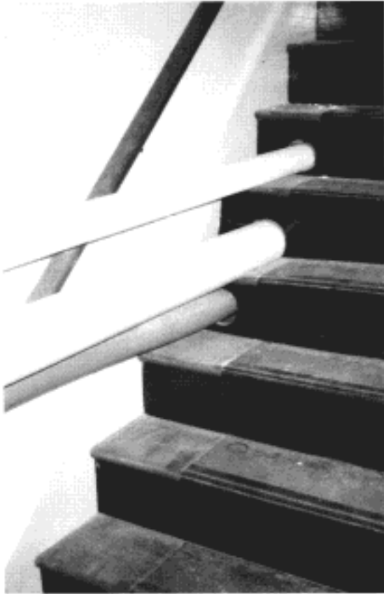
Mid-twentieth century West Lawn heating main and electrical service
