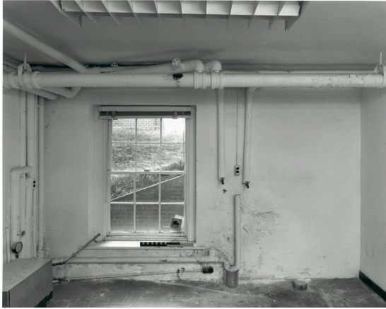
Laundry Room B02
