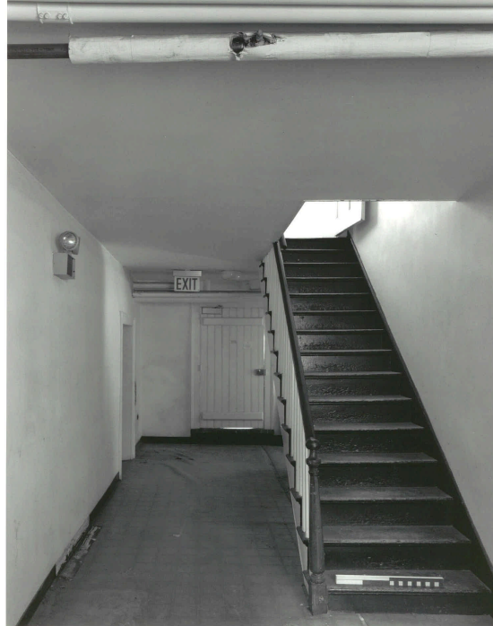
Stair Hall Room B06
