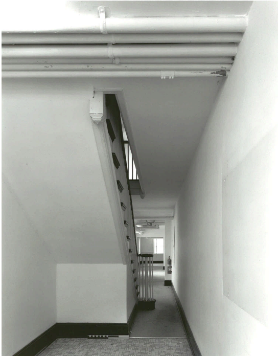
Stair Hall Room B10
