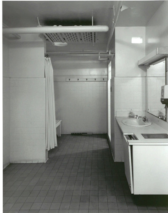
Men's Restroom B08
