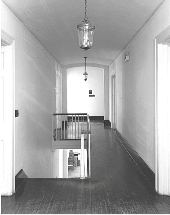
Back Stair Hall, Room 106
