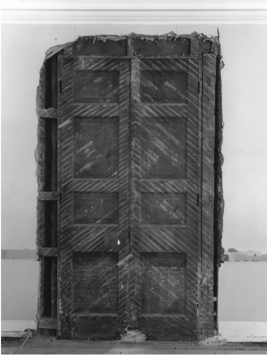
East Elevation door uncovered, Room 102
