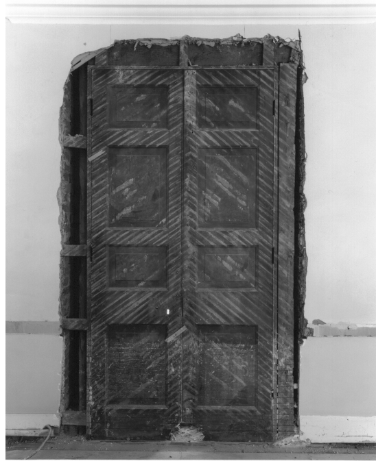
Original entry door to Room 102 during excavation work
