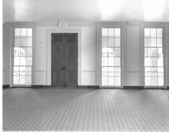
East wall of Room 102
